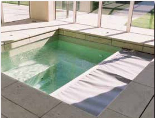
RECESSED UNDER TRACK ON AN INDOOR INGROUND SPA
